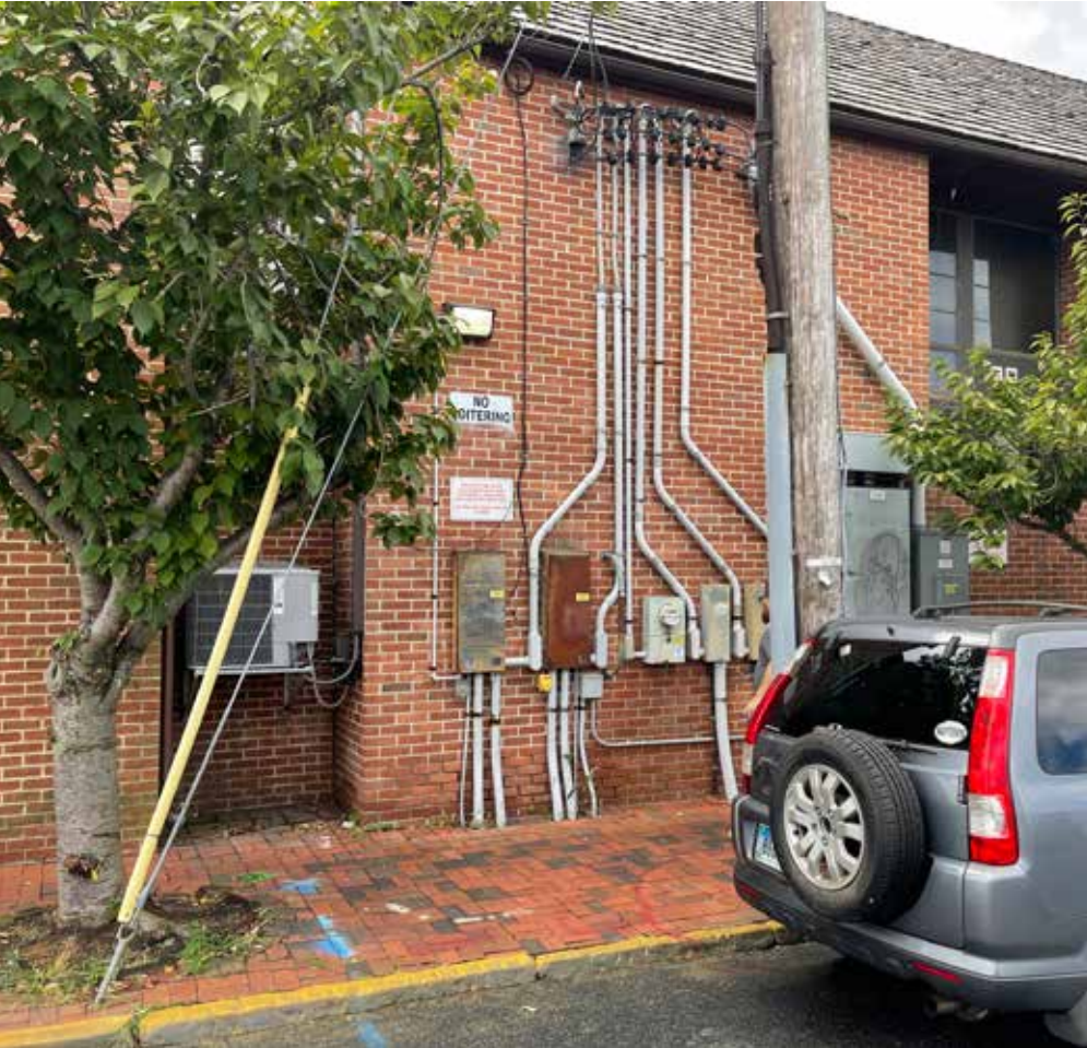
Existing Electrical Service Equipment on Harbormaster Office
